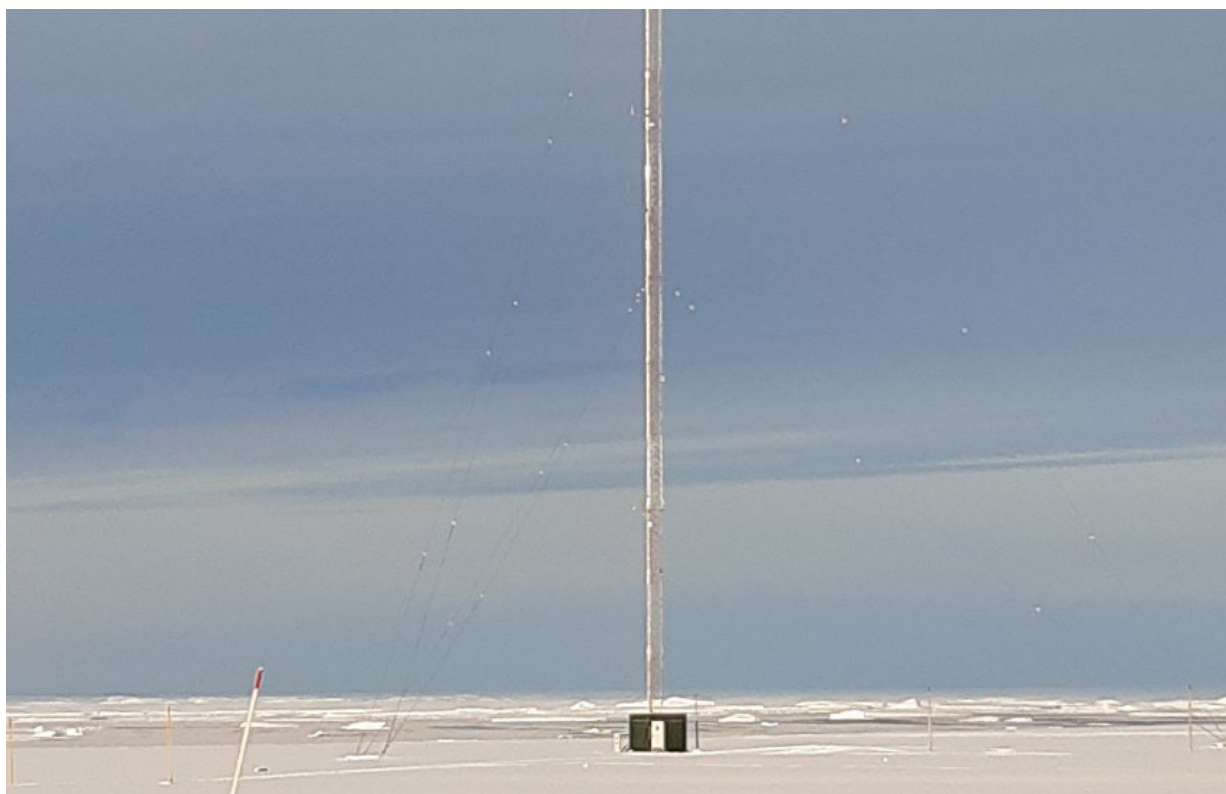
Figure 2.1. ICOS-SNO at Villum Research Station, Station Nord
